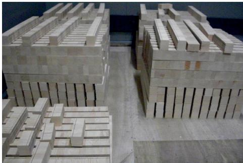
**Do not install unless heating, air conditioning, and humidity controls are in full operation and room conditions are normal.** Prefinished End Grain Blocks are available in strips  $\frac{3}{4}$ " and 1" depth, kiln-dried to 6-8%. All flooring strips must be allowed to adjust to your specific room condition. Only after HVAC systems are operating normally and assuming a room temperature between 65° and 75°, remove packaging and space strips apart so that the air reaches both top and bottom
